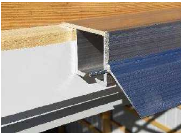
21. Install Ultra Glide Track. Face-mount or top mount is relatively the same; face mount uses 2 locking pins vs top mount has 1. Face mount is 1" shorter clearance on door leaf height
