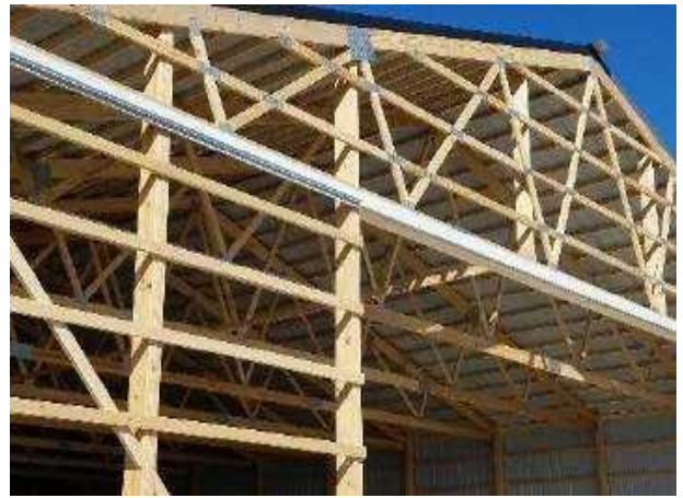
20. Install track board trim, covers underside of track. This is not crucial but these are premium doors going on premium buildings. Exposed wood is not premium
