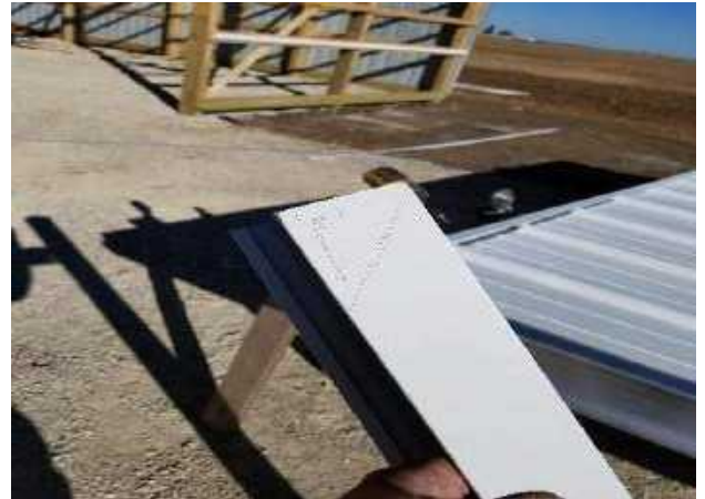
15. Back side top of vertical frame cover needs to be cut at an angle 3" so trim doesn't catch header. Bottom inside of vertical frame cover needs to be notched slightly to fit over B1
