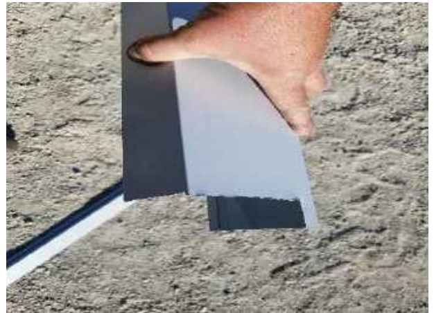
14. Install vertical frame cover. Inside & bottom gets notched 4 1/4" x 1" to go around bottom C on jamb end and to accept center guide. Cut flush with top of door, fasten at bottom, top, and at each girt. Install "T" trim on prevailing wind door panel.
