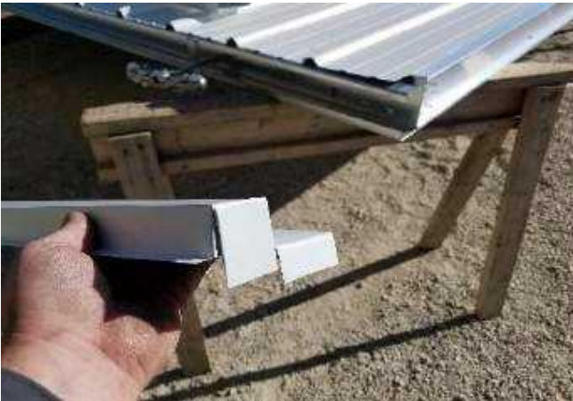
16. Fold down ends of hat trim to cap door. Do not screw tabs on ends. Notch around trolleys.
