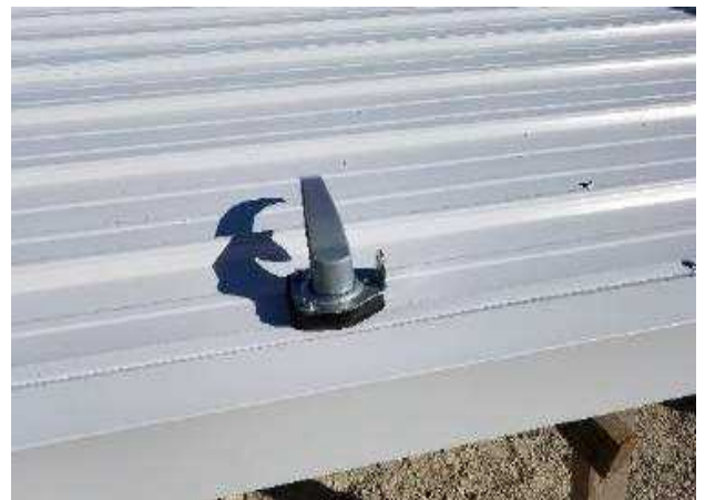
18. Install exterior handle with rubber gasket against steel and plastic filler plate; fasten with 3) 12 x 1.5" screws. Make sure handle is centered and square. Handle can be inserted 4 directions, make sure the "neutral" position is down, between rod up and down.
