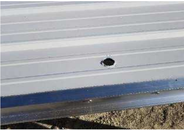
13. Drill and cut hole for exterior handle through steel.
